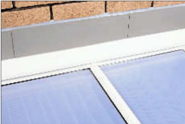
1.12 Conservaflash may also be used on extensions where the floor area does not exceed 30 m<sup>2</sup>, given the appropriate soaker detail. However this use is outside the scope of this Detail Sheet.
