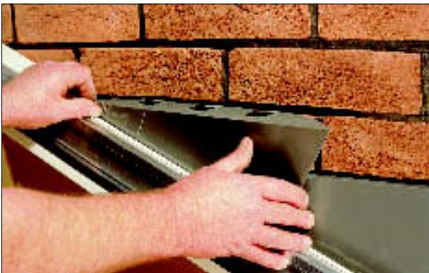
9.17 For duo-pitched roofs the saddle apron panel and horizontal flashing is installed at the ridge and the joints are sealed with silicone.
