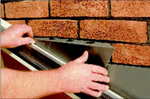
9.17 For duo-pitched roofs the saddle apron panel and horizontal flashing is installed at the ridge and the joints are sealed with silicone.
