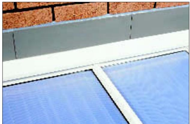
1.12 Conservafash may also be used on extensions where the floor area does not exceed 30 m<sup>2</sup>, given the appropriate soaker detail. However this use is outside the scope of this Detail Sheet.
